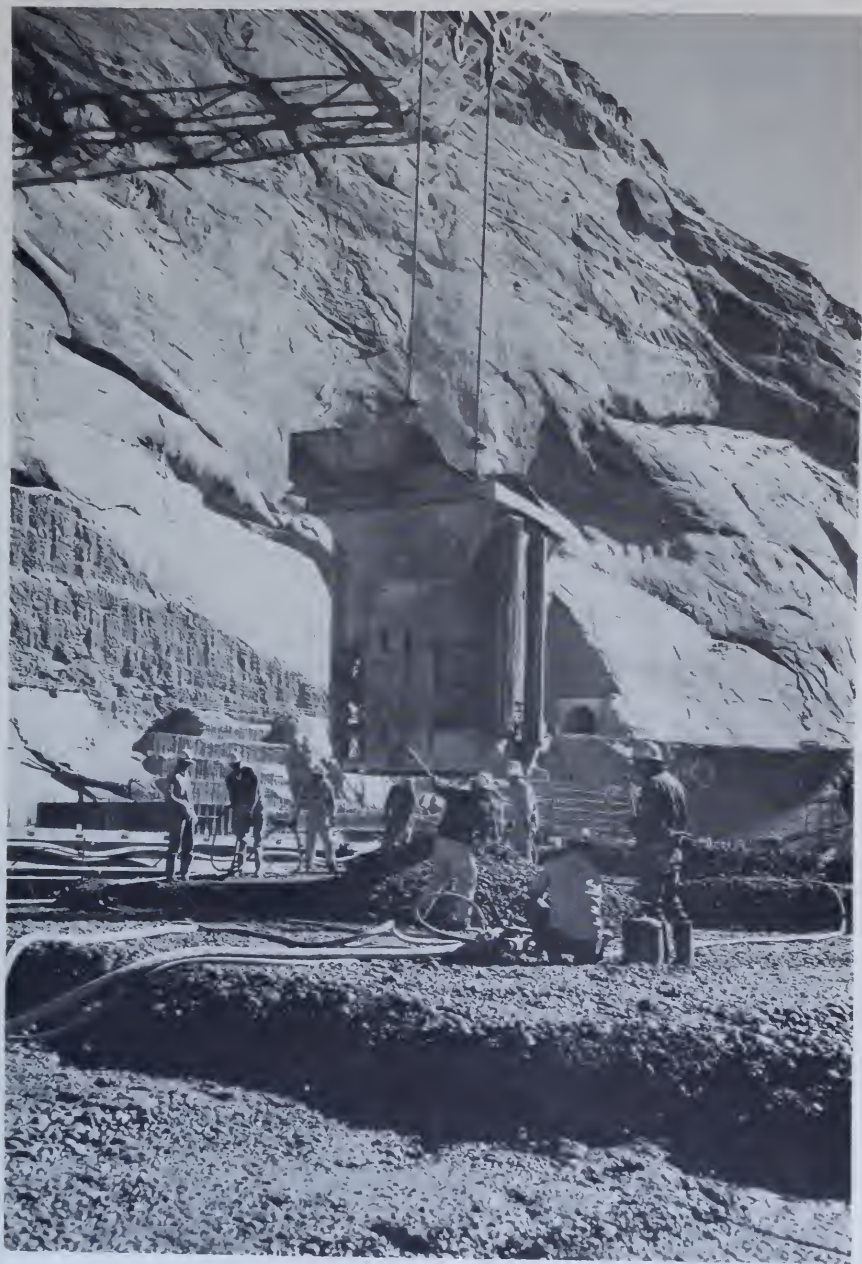
Figure 130.—A 12-cubic-yard bucket which will readily discharge concrete of low slump, permit slow or partial discharge, and dump the concrete in relatively low twin piles requiring a minimum of lateral movement during consolidation. P557-420-05480.
